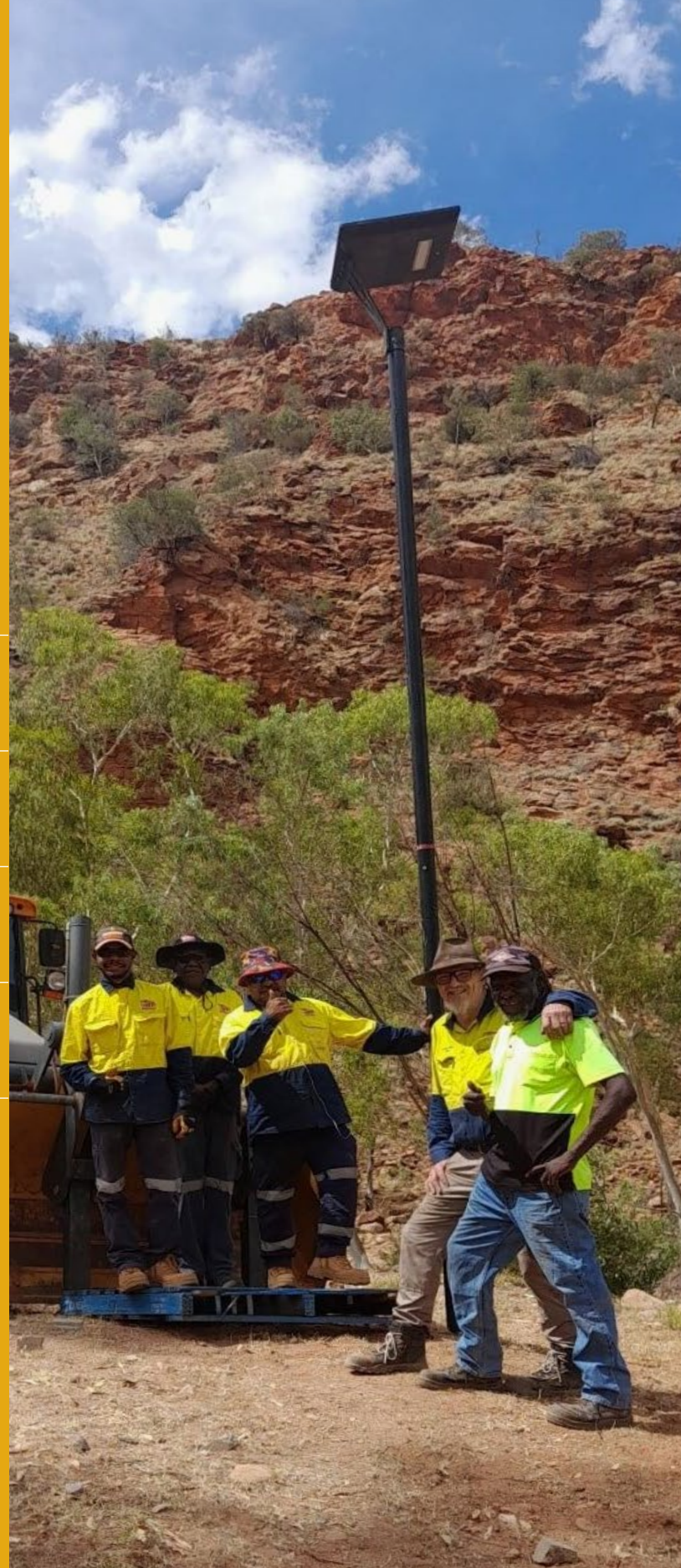
Areyonga Team installing solar lights
