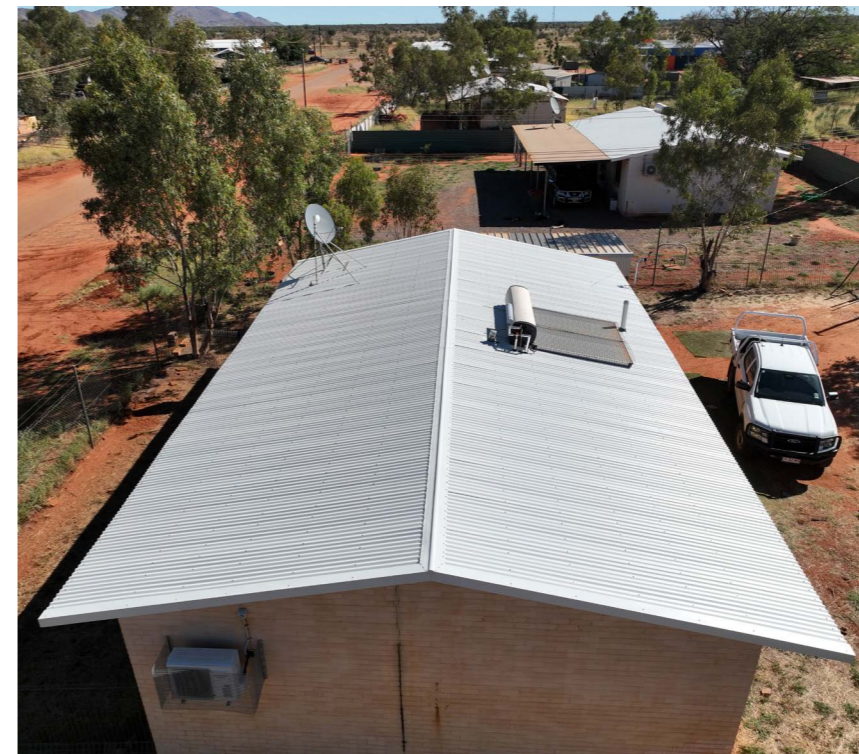
Lot 248 Papunya - staff house new roof cladding
