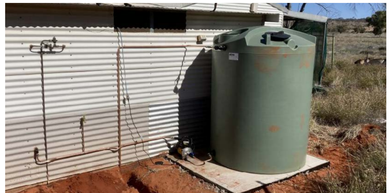
John Holland - Supply and installation of pressure pump and creak tanks
