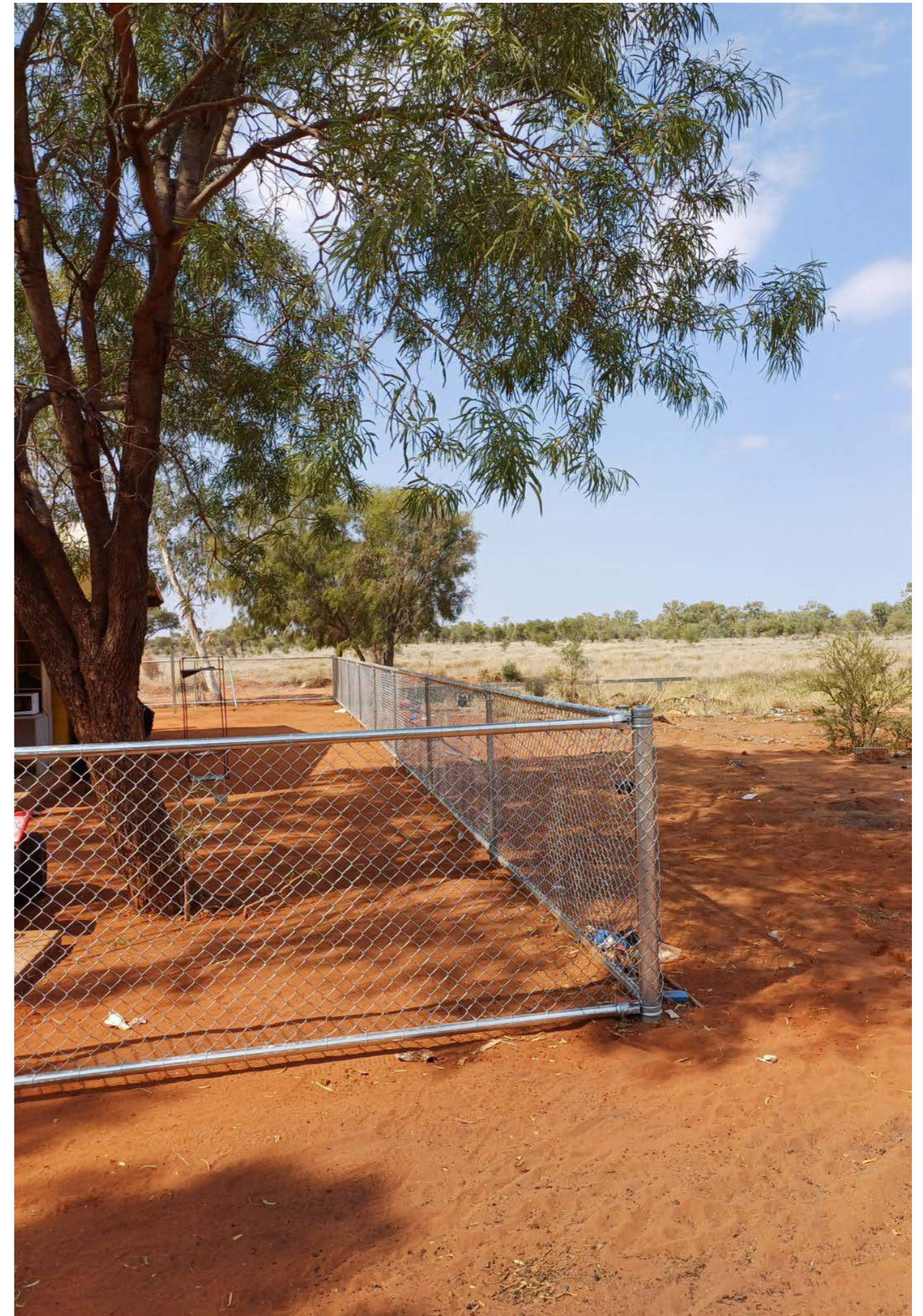
Installation of new fencing for the houses at M'Bunghara Outstation
