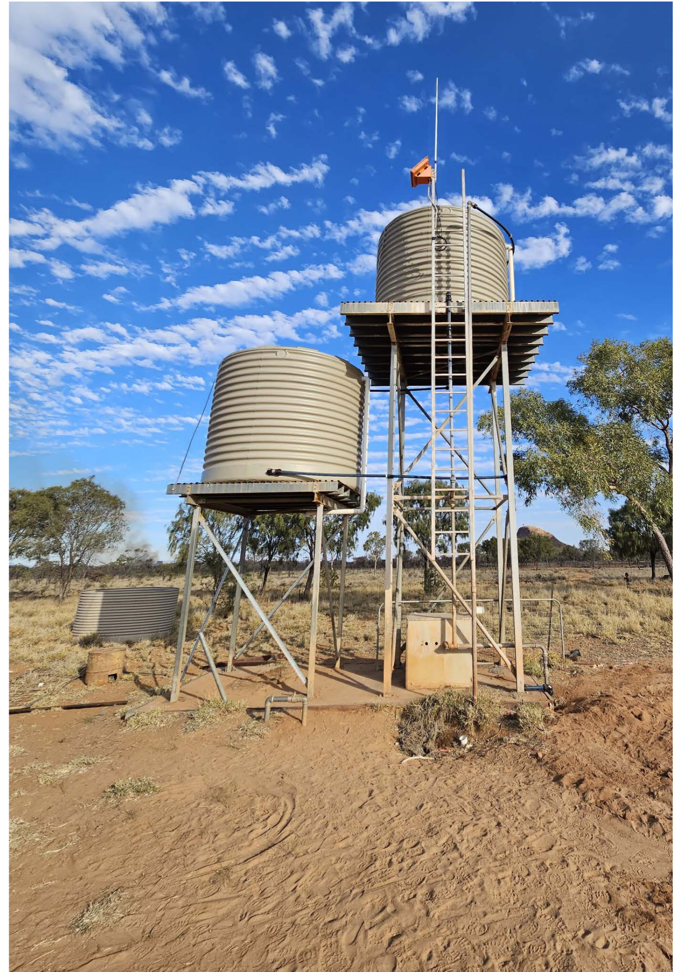
| Atji Creek – Supply and installation of fencing and poly water tank
