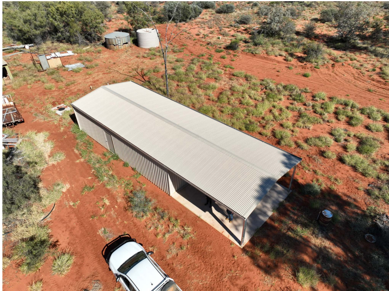
| West Waterhouse – Supply and installation of structure
