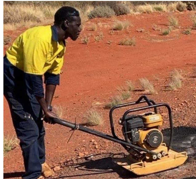
Patching the roads in Kintore
