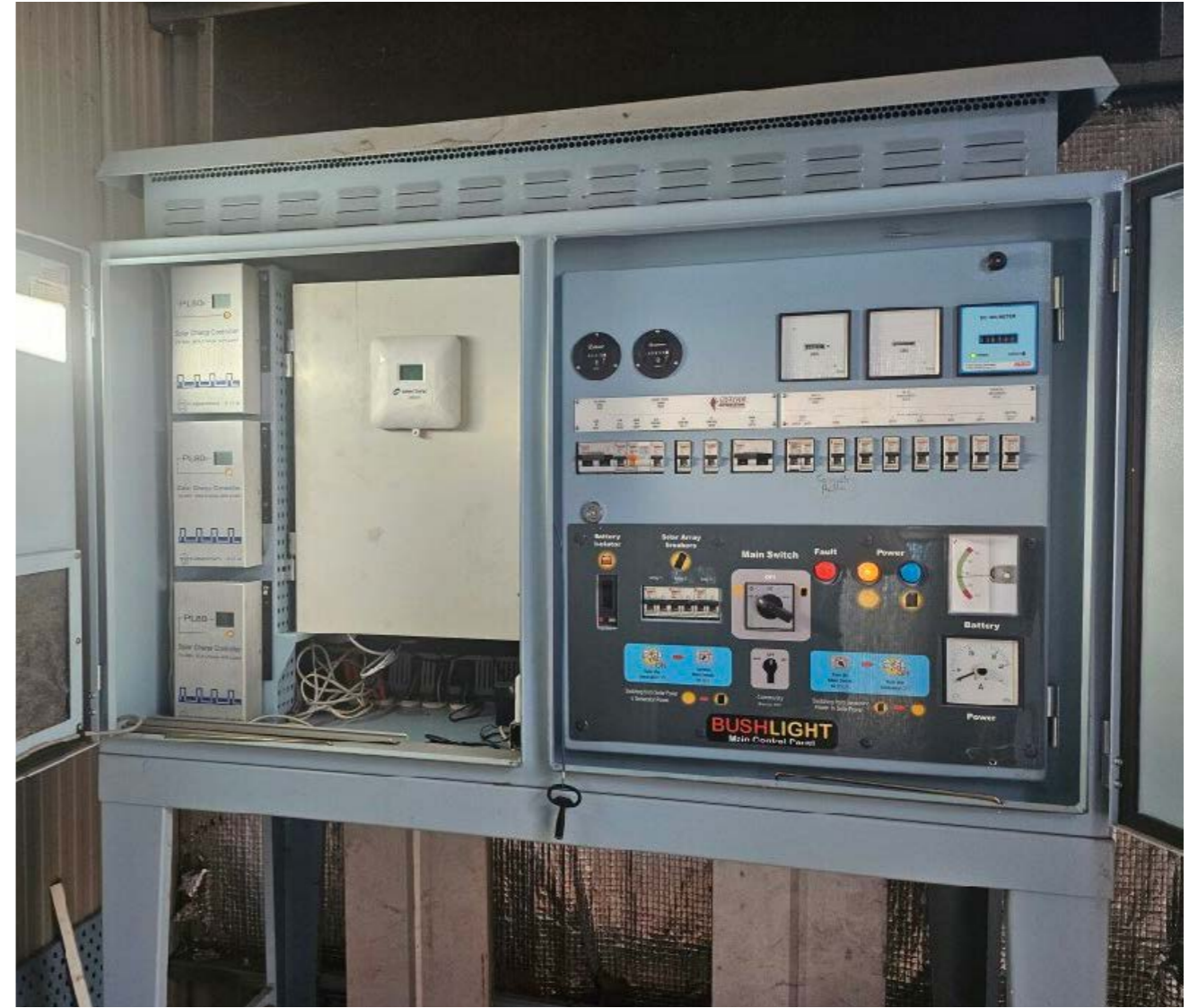
Warren Creek - Supply and installation of new solar power system
