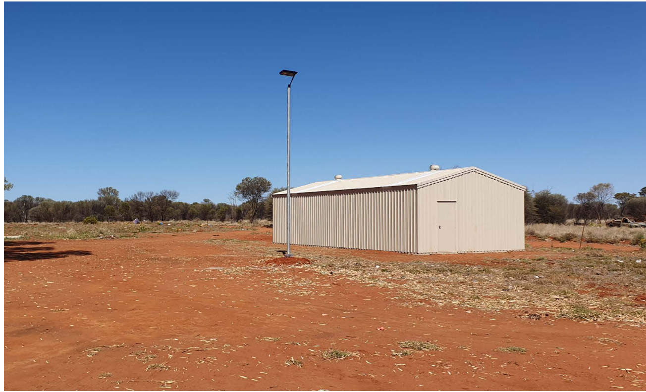
| Ngankiritja – Supply and installation of shed and solar lights
