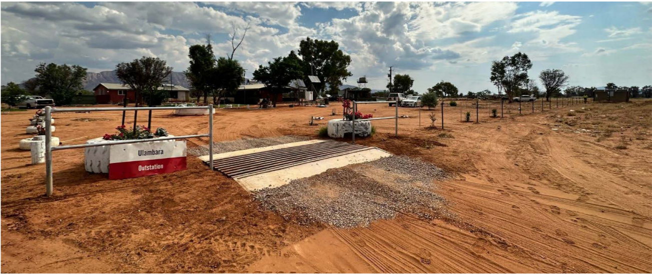
Ulambara - Supply and installation of cattle yard, fencing and grid
