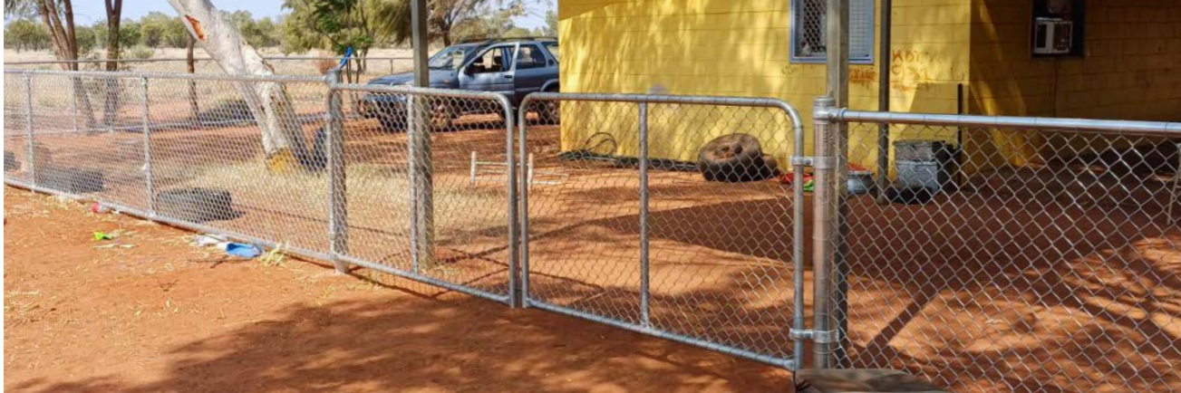
M'Bunghara - Supply and installation of fencing at 6 properties
