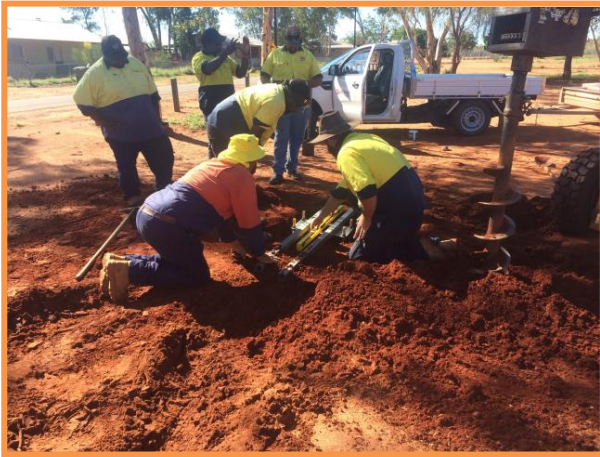
Installing footing for Solar Lights
