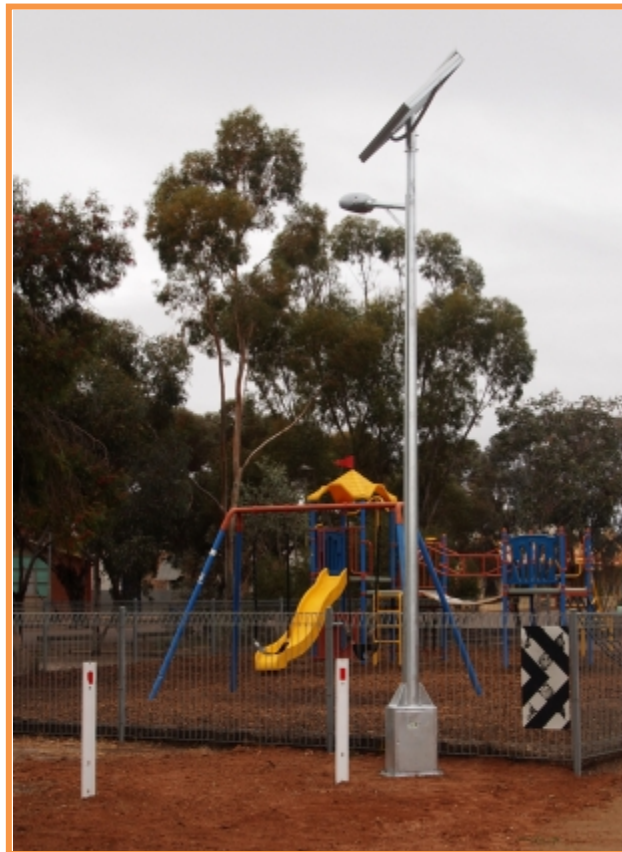
Example of what the lights will look like when completed
