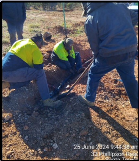
Repairing Water leaks
