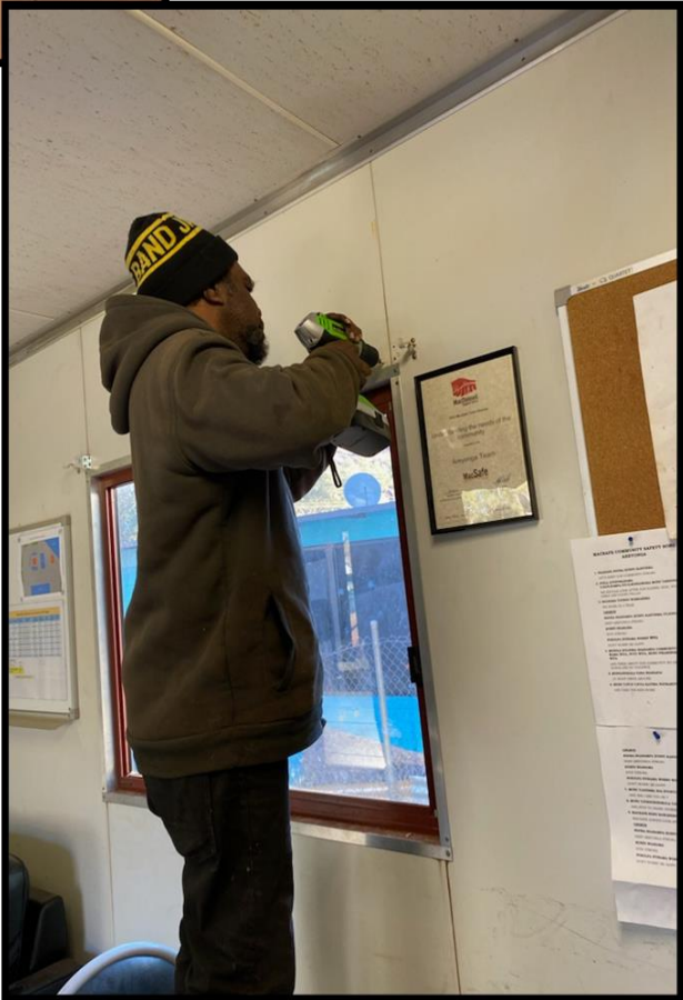
Wilbur installing the new blinds in the MacSafe office.
