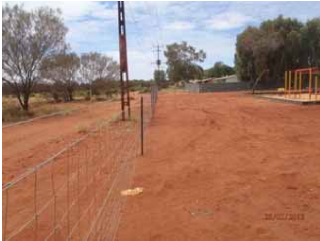
Back fence completed at L Penham Park
