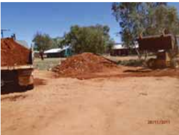
Civil Works at Haast's Bluff
