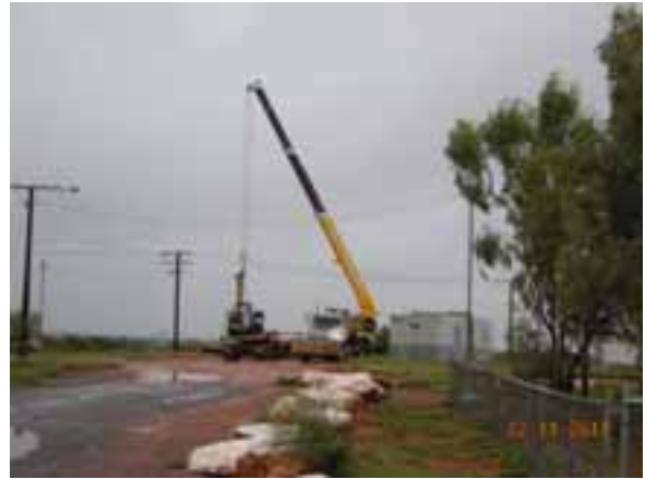
Road works at Imanpa
