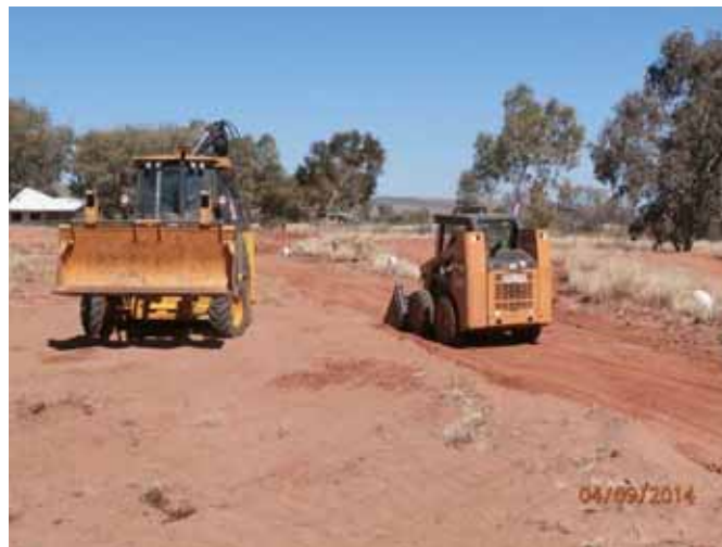
Preparing the running track for the SmartStart project
